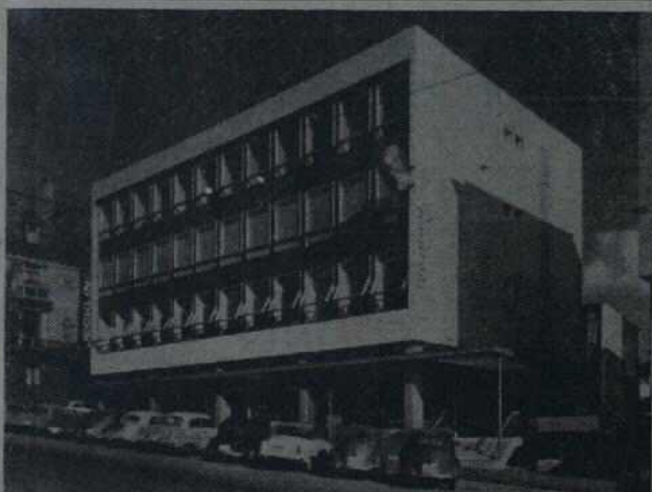
Storefront of Jecklin Music Shop, Zurich, Switzerland. Ground floor and basement are devoted to disk sales. Front and sides are entirely glass, leaving an unobstructed view of promotions, displays and equipment for passers-by.
