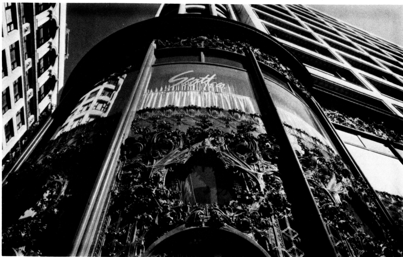
Carson Pirie Scott & Co.'s ornate wrought iron entrance facade at 1 South State Street is a Chicago landmark. It was designed by Louis H. Sullivan and completed in 1904 and is just one example of the Chicago School of Architecture.
