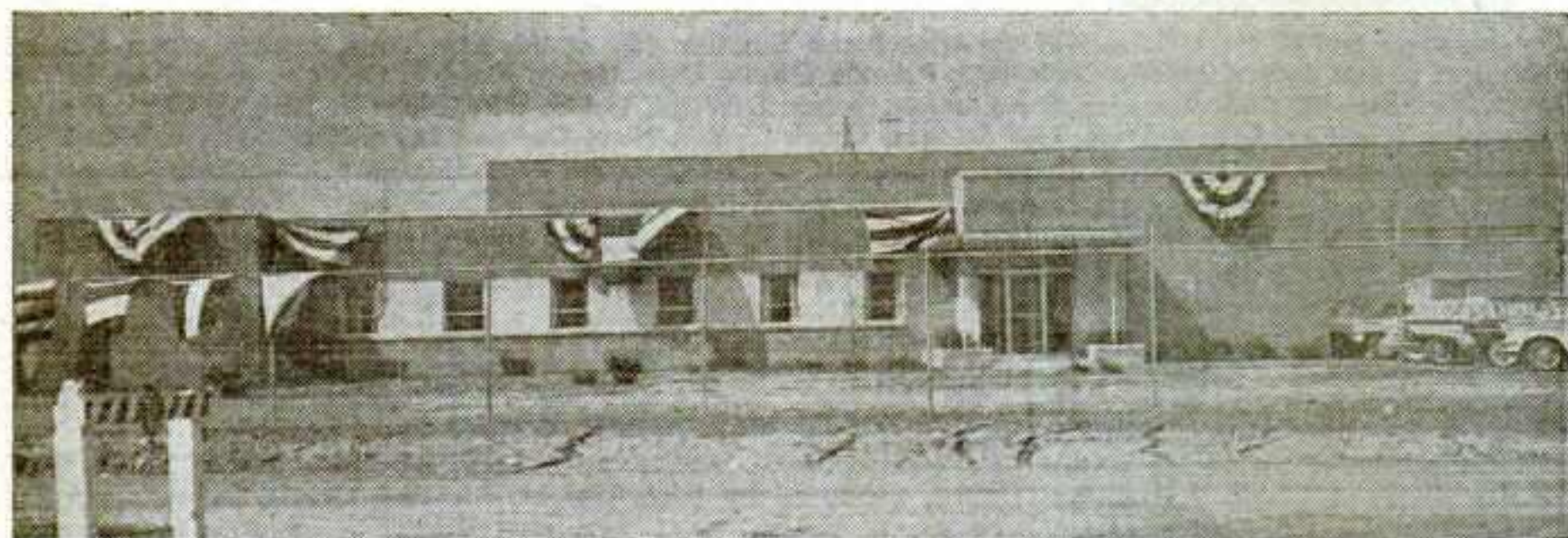
Front and sides of the office section of the combined office-factory are of enameled-face brick. Exterior of remaining portion of the huge structure is of concrete block. The entire 10-acre plant is fenced with a seven-foot-high chain link fence, topped by three strands of barbed wire.
