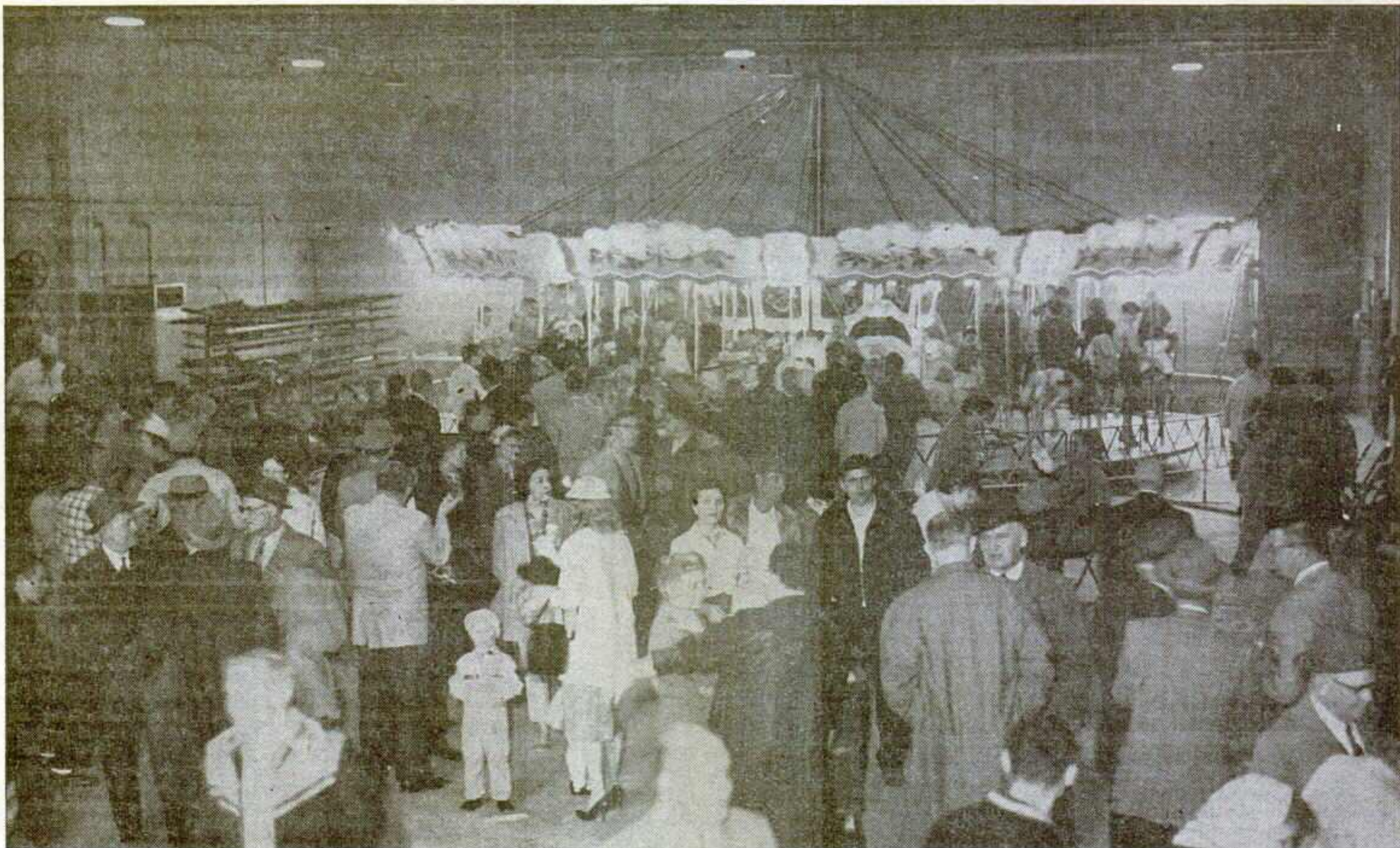
Guests at the open house Saturday (9) at the new Columbus, O., factory-winter quarters and offices of the Gooding Amusement Company were impressed at the size and facilities of the plant. An idea of the size is given by the machinery shop, a 65 by 125-foot section, shown above during the open house. The Merry-Go-Round, in operation at open house to the delight of youngsters, looked as tho it had just come, brand new, out of the factory. Actually, the device, built by Allan Herschell Company, was used for the first time in 1934 at the Great Lakes Exposition, Cleveland, and has been put up and torn down at least 600 times since. Its sparkling appearance and smooth operation is a testimonial to the craftsmanship of the Gooding winter quarters-factory personnel.
