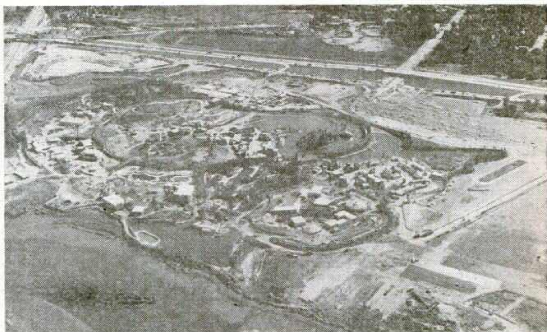
FREEDOMLAND, NEW MAJOR NEW YORK-THHEME PARK, opens to the public on Sunday (19) at the peak of a publicity and advertising blast in all media. Seen from the air, the site adheres to the general contours of the United States. At upper left is a semi-circular foundation of a motel. Parking area is at lower right. Landmarks visible here include the Great Lakes, Gulf of Mexico, South Texas and the West Coast. The 41 theme sights and rides are located according to geographical connections. Construction is proceeding in many areas, including the Florida peninsula.
