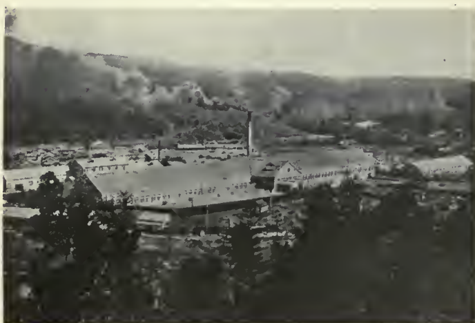
THE ELECTRIC REFINERY OF THE HITACHI MINE.
