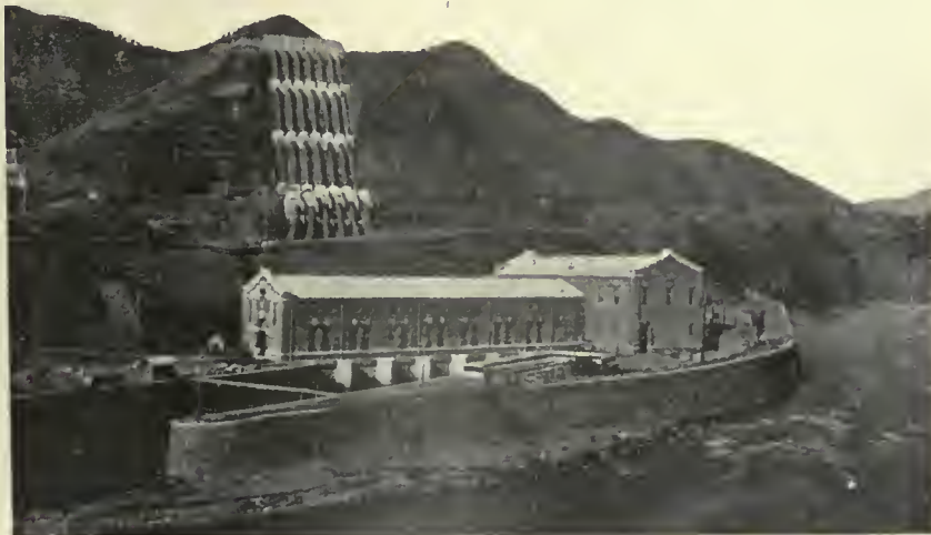
THE KOMABASHI POWER STATION.
