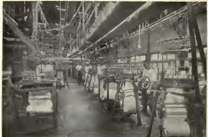
INTERIOR OF THE FACTORY.
