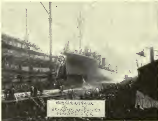
THE DESTROYER "HAMAKAZE" PAINTED WITH TALLOW MANUFACTURED BY THE CO.
