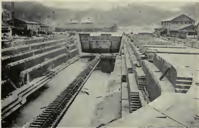
DOCK, LENGTH 500 FEET, MAIN WORKSHOP.
