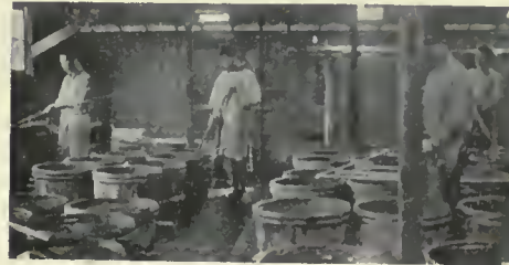
(2). INTERIOR OF THE WORK.
