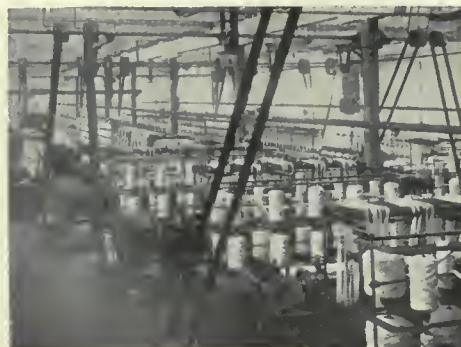
INTERIOR OF THE WORKS.
