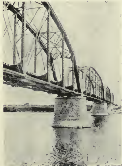
AGANO IRON BRIDGE ON THE SHIBATA LINE.
