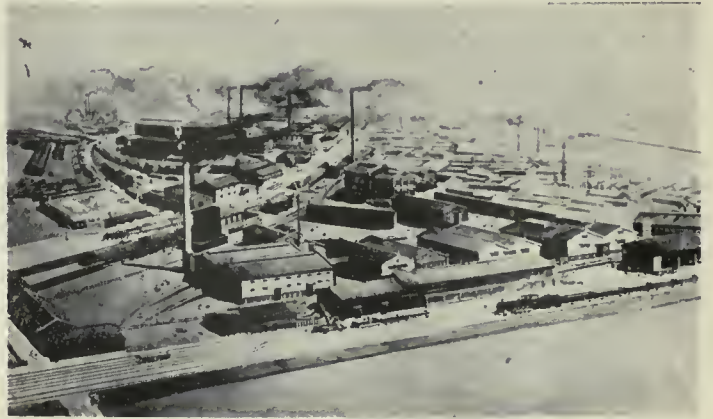
TOKYO FACTORY OF THE SHINAGAWA WHITE BRICK CO.
