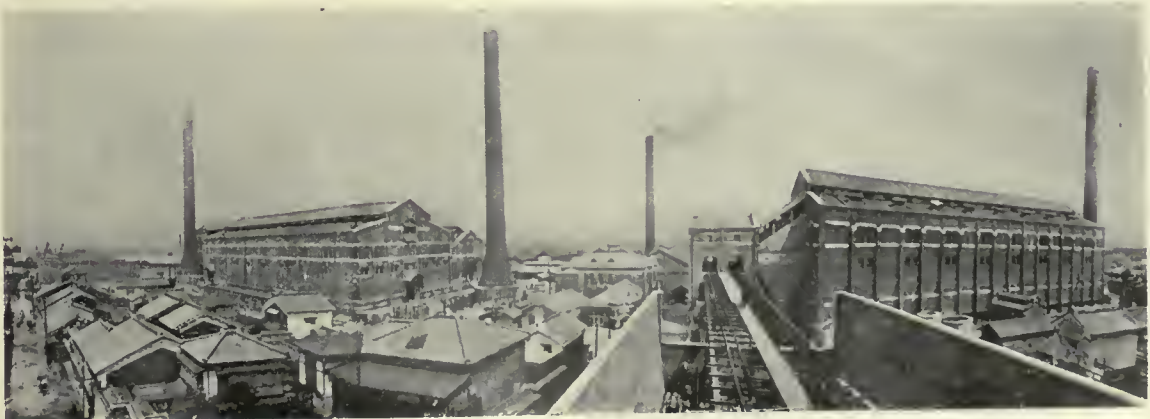
AJIKAWA POWER HOUSE OF THE OSAKA ELECTRIC LIGHT CO.
