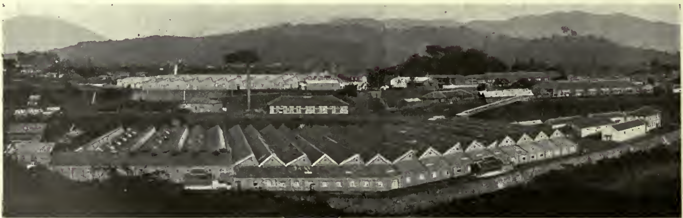
PART OF THE OYAMA WORKS OF THE FUJIGASU SPINNING CO.
