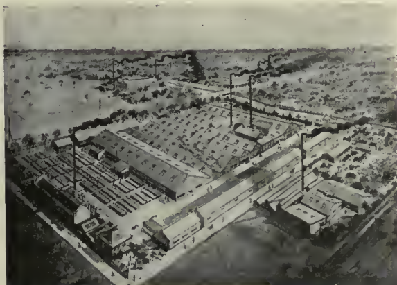
TOKYO FACTORY OF THE NIPPON PAINT MANUFACTURING CO.
