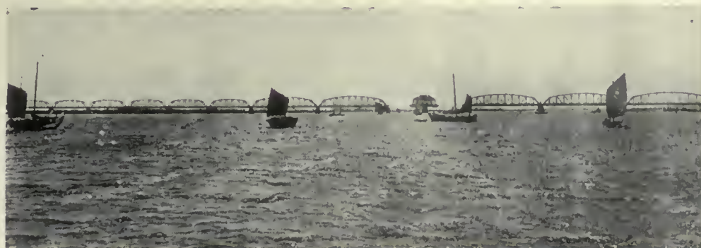
RAILWAY BRIDGE OVER THE YALU RIVER.
