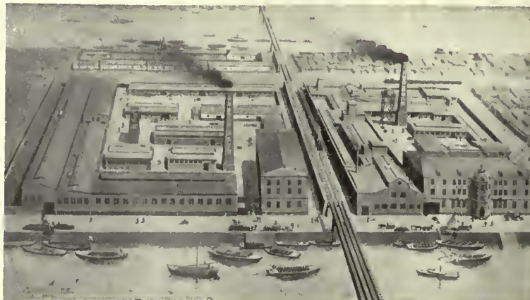
THE ITO ACETIC AND CHEMICAL WORKS, OSAKA.
