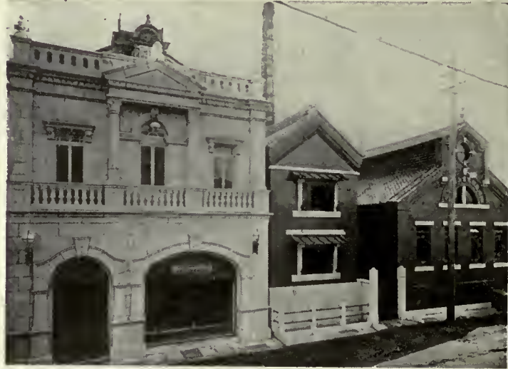
HEAD OFFICE OF Y. TOMIYAMA & CO., TOKYO.
