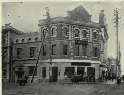
THE BUSINESS OFFICE IN KYOBASHI, TOKYO.
