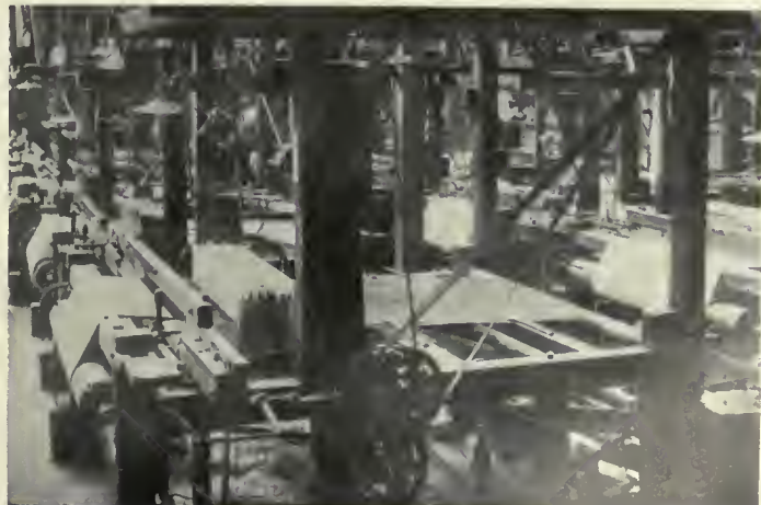
INTERIOR OF THE FACTORY.
