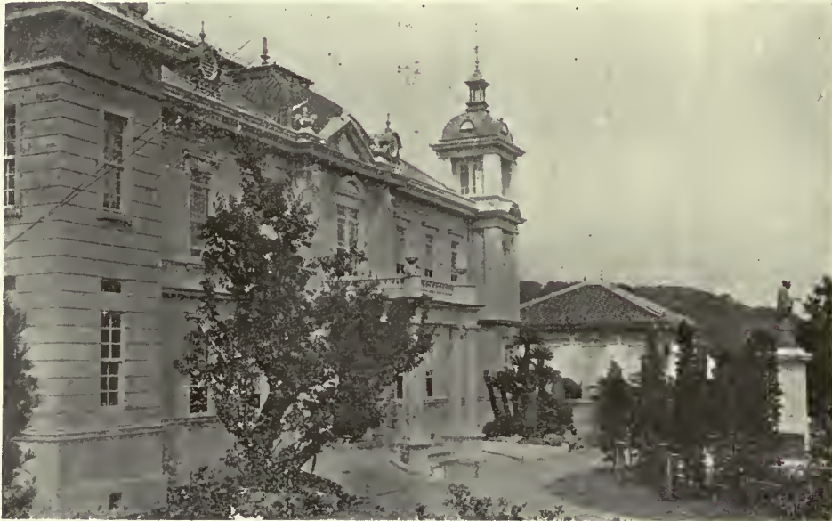
THE BUSINESS OFFICE OF THE YOKOYAMA MINING DEPARTMENT.
