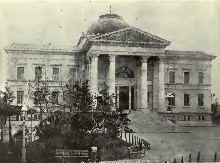
THE OSAKA PREFECTURAL LIBRARY.
