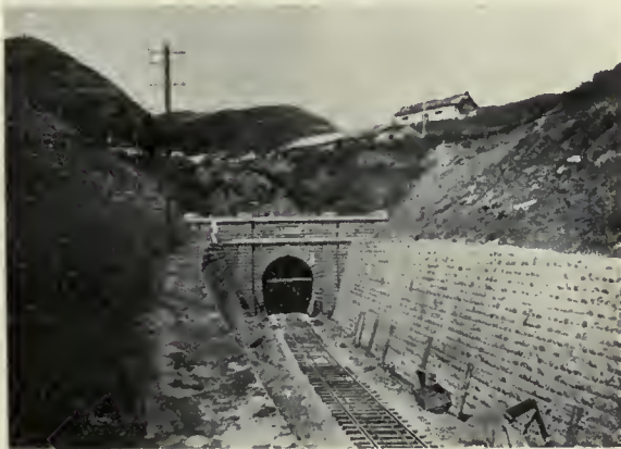
THE FUCHINANG TUNNEL ON THE ANTUNG-MUKDEN LINE.
