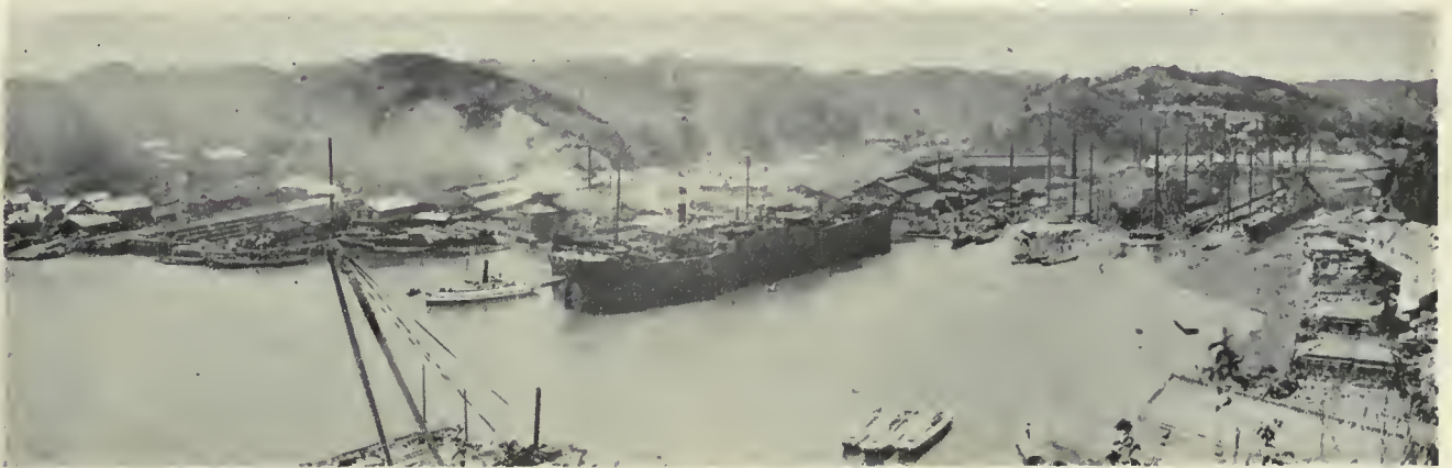
MAIN WORKS OF THE URAGA DOCK CO..
