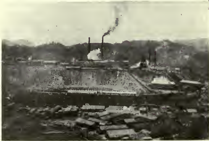
MACHIDA SHAFT AT UCHIGO MINE.
