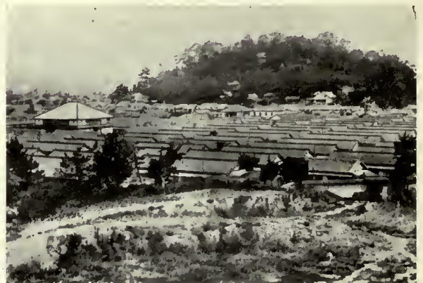
THE BOARDING-HOUSE FOR WOMEN OF THE KURASHIKI WORKS.
