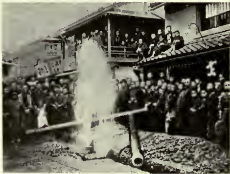
EXPERIMENT WITH WOODEN PIPES LAID BY THE COMPANY IN MATSUMOTO.
