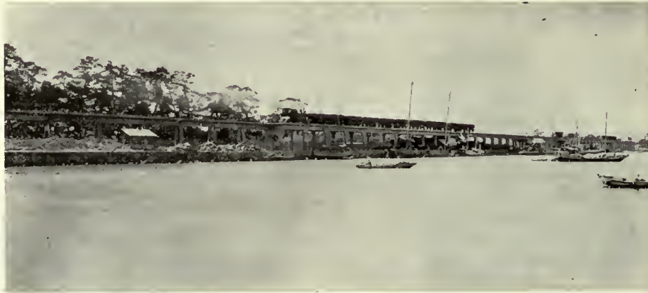
RAILWAY BRIDGE OF THE KOKURA RAILWAY CO.
