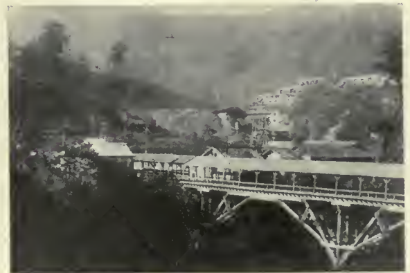
SHINYUBARI MINING OFFICE AND ITS ENVIRONS, HOKKAIDO.
