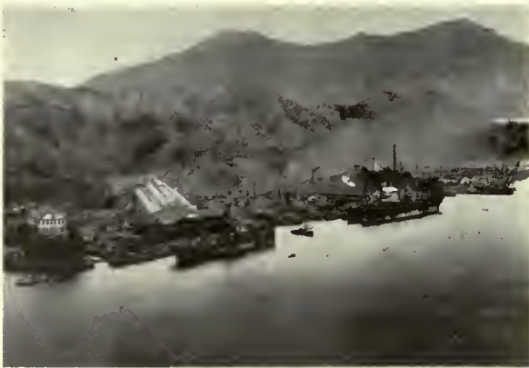
INNOSHIMA WORKS OF THE OSAKA IRON WORKS.
