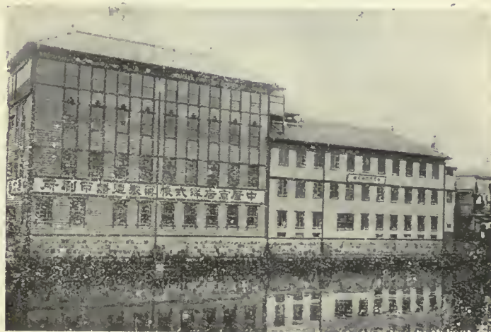
THE NAKAYA PRINTING HOUSE, TOKYO.
