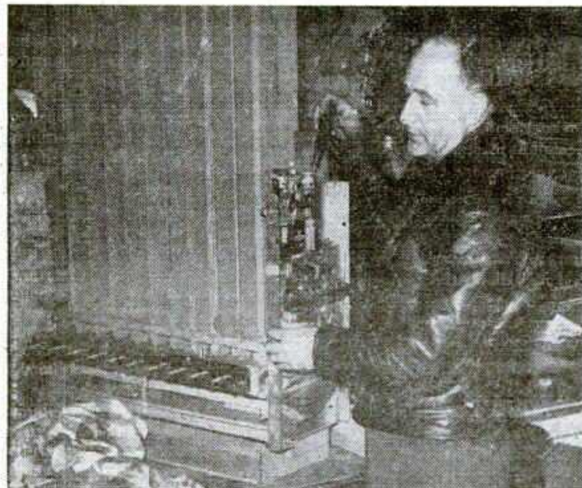
CANDY MACHINES OPERATED by Aaron Strouse are regularly pulled in to his shop for servicing and routine maintenance. Here Strouse adjusts the coin mechanism on an overhauled multi-column venter.
