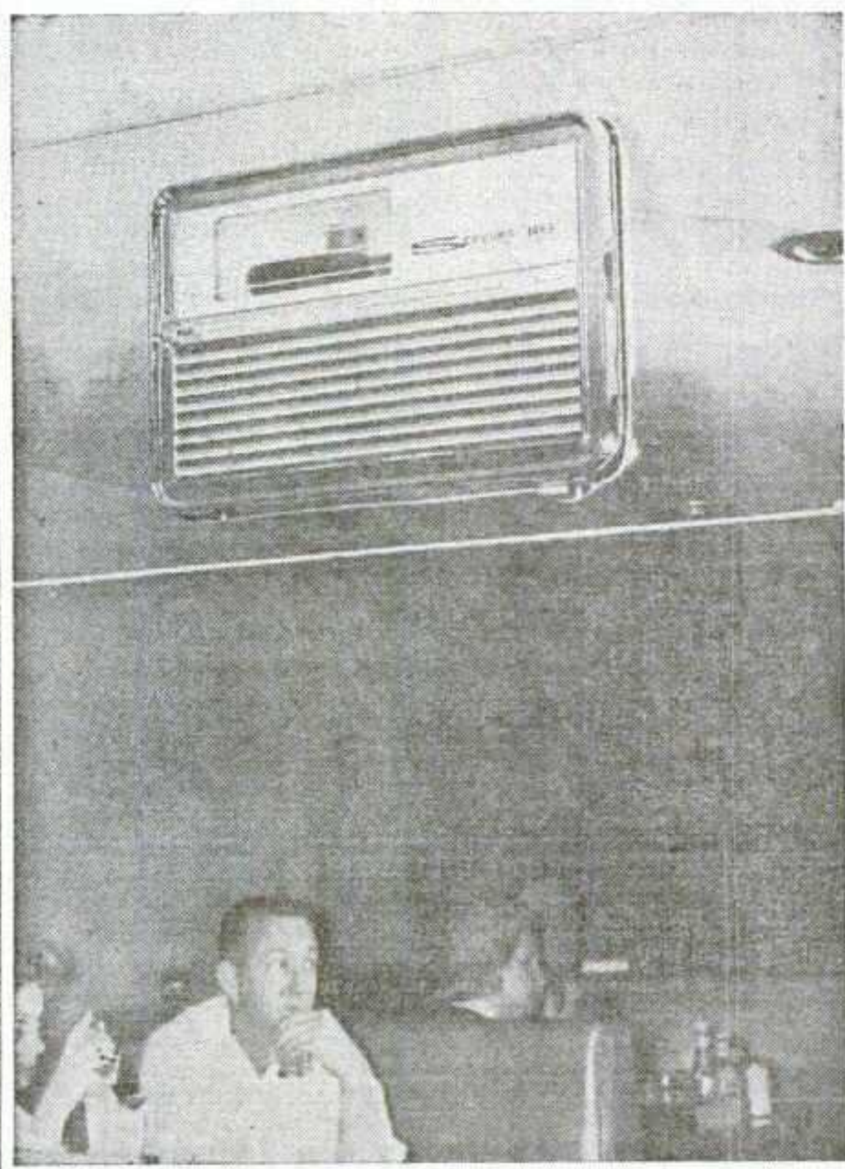
EFFECTIVE DISPLAY: A glasscutter was employed to cut a rectangle thru a mirror mounted on one wall of Phoenix's New Yorker Bar, and a 1,000-selection background music unit was installed in the mirror.
