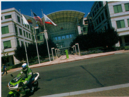
Research and Development building 1 at the Apple corporate headquarters in Cupertino, CA. Apple spends a significantly larger portion of its income on R&D than most high-tech companies
